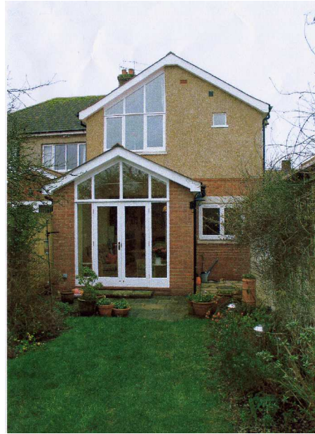
Rear Elevation, after
